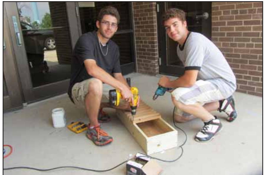
Brian and Addison are working on building projects with Mr. Schultz
